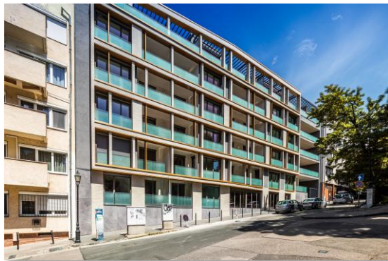
Naphegy 12 Budapest completion in 2024 42 units
