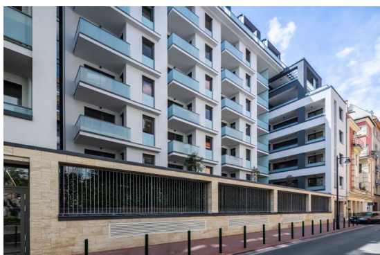
Corvin Next Budapest completion in 1H2025 100 units
